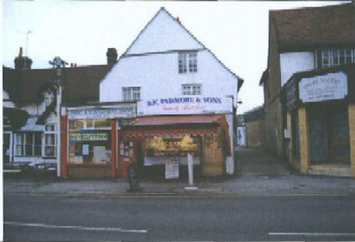
Access off High Street
